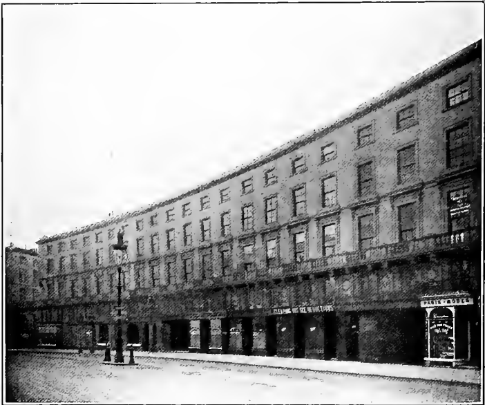
Site of The Piccadilly Hotel before demolition of houses in 1906
